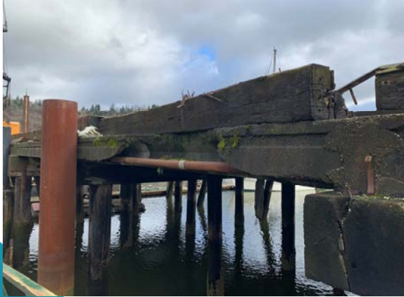
Decking Damage
