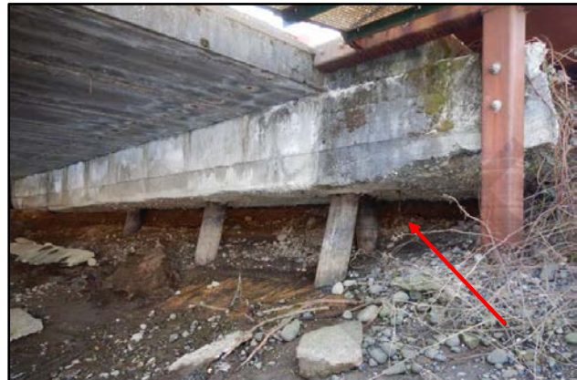
Abutment Erosion
